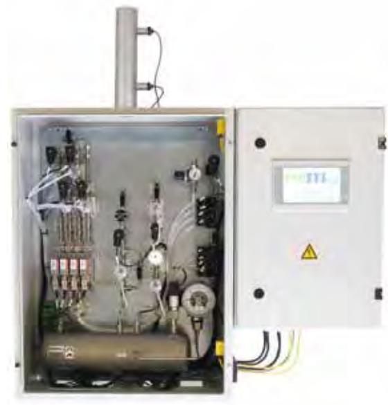
Example of a complete system including safety device in ATEX Zone II
